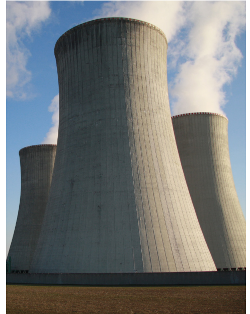
Figure 1. Cooling towers at a nuclear power plant
